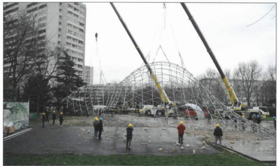
Fig. 7: Grid during erection
