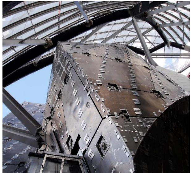
Figure 9: Aluminium support shell for Ductal panels
