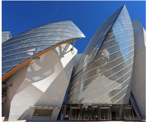
Figure 7: Iceberg cladding at entrancePrimary
